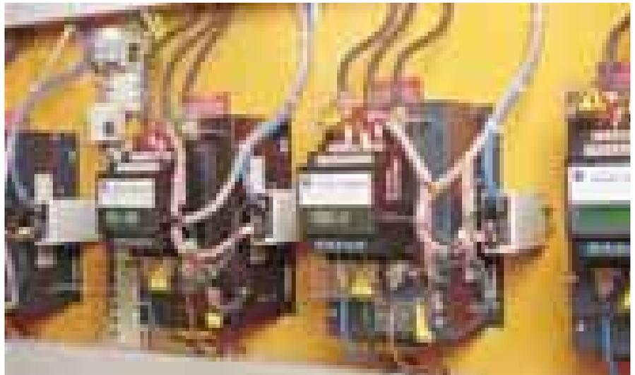
*Every water pump is controlled by its own SMC Dialog Plus soft starter. The function "pump control" fulfills all the requirements of an optimum drive.*
