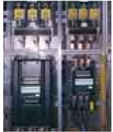
*The “Pump control” mode on the soft starter SMC Dialog Plus provides unique interactive control that reduces the pressure waves in centrifugal pumps. Although smoothness of control is similar to a regulator, a speed transmitter is not required on the pump motor.*
