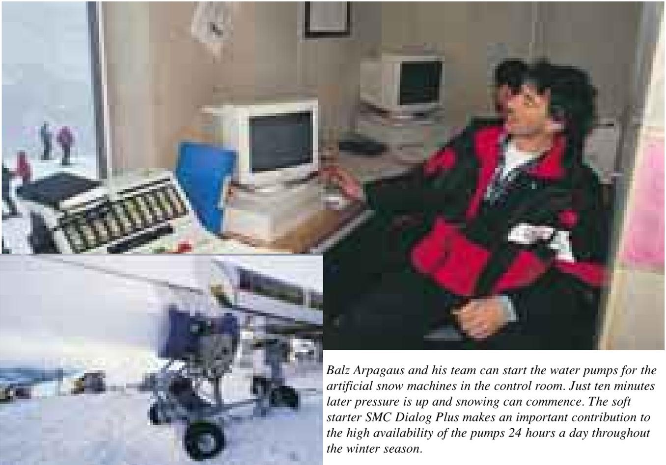
*Balz Arpagaus and his team can start the water pumps for the artificial snow machines in the control room. Just ten minutes later pressure is up and snowing can commence. The soft starter SMC Dialog Plus makes an important contribution to the high availability of the pumps 24 hours a day throughout the winter season.*
