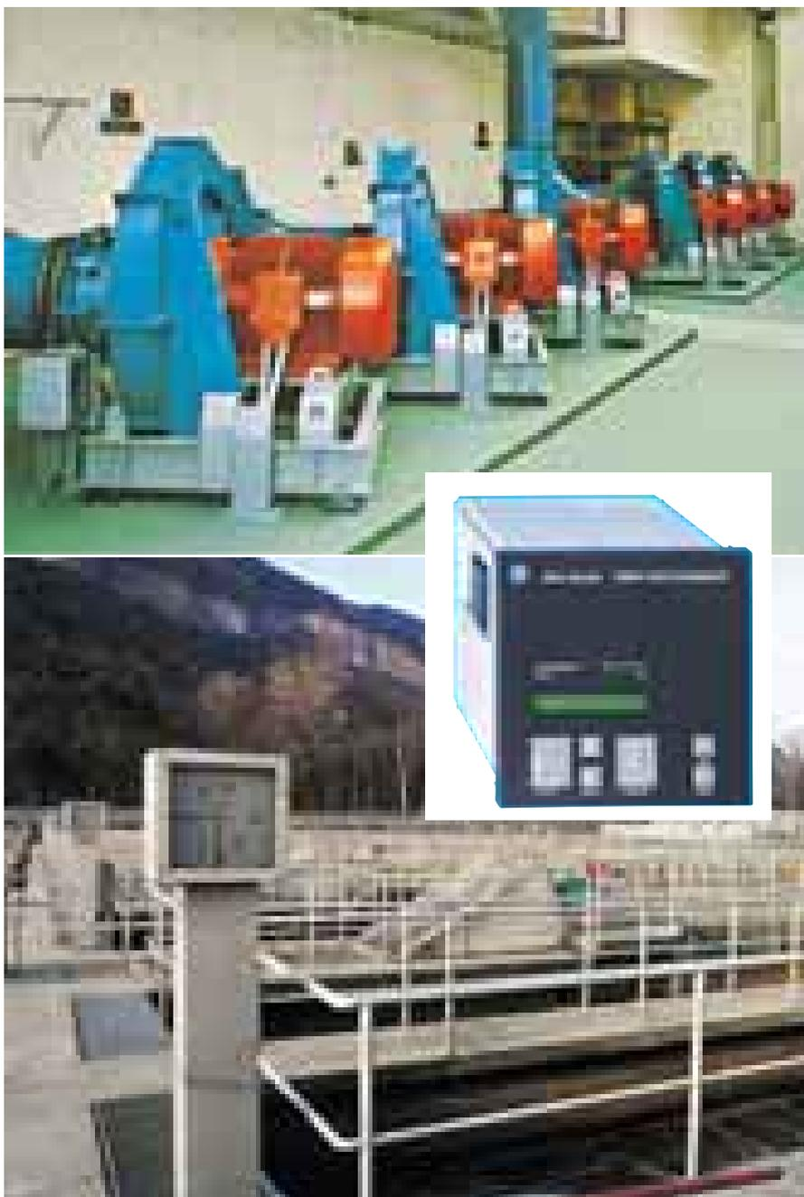
*The three fans each with a rating of 75 kW are arranged physically in series and starting and operating them in cascade was critical. The problems were solved by installing the electronic control and protection system of the 825 series which achieves maximum utilisation without risk to the motor by forming a thermal image of the conditions in the motor.*
