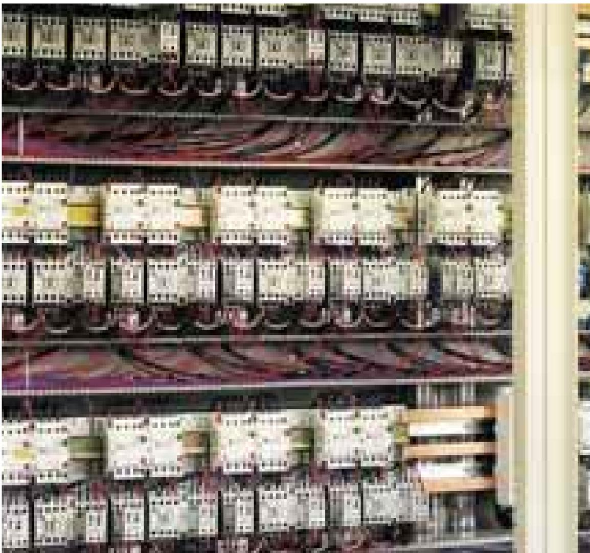
*View inside the switchgear cubicle at the waste water treatment plant: the Modular Control System (MSC) was the first choice for compact well designed power feeders.*
