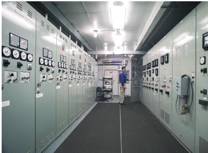
**The Rockwell Automation Power & Energy Management Solution installed at GlaxoSmithKline's Collegeville research facility monitors incoming power for level fluctuations and in the event of a power loss, the system re-powers the facility using onsite power generation capabilities.**
