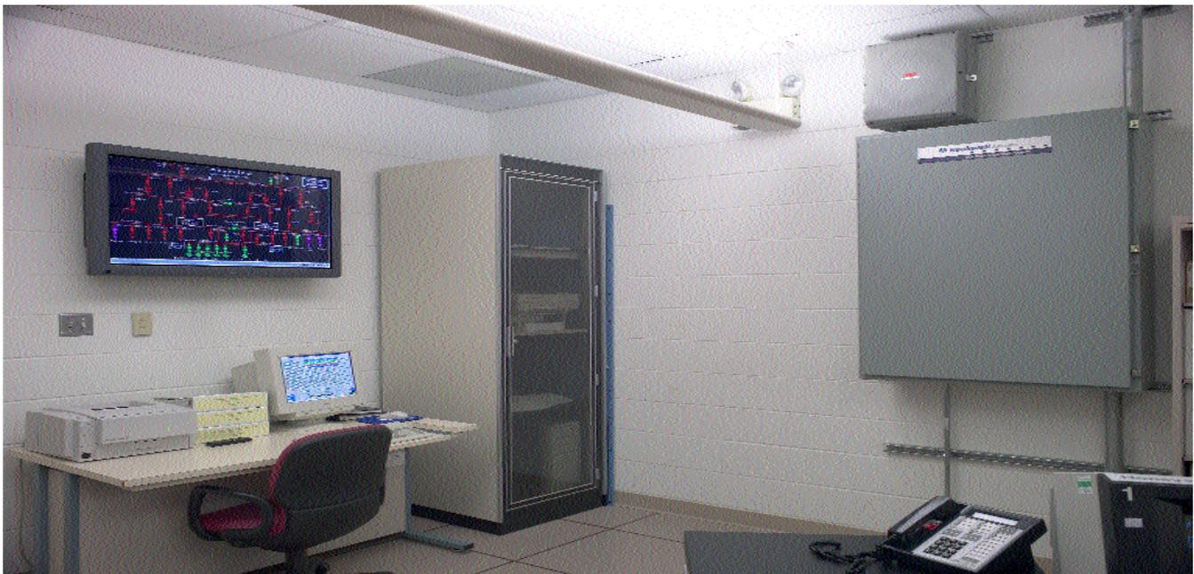
***Data gathered from the substations and incoming utility power lines is graphically represented using Rockwell Software RSView32 visualization software displayed on a large flat panel monitor. The system allows operators to quickly survey system status and the effects of transitioning to emergency power.***
