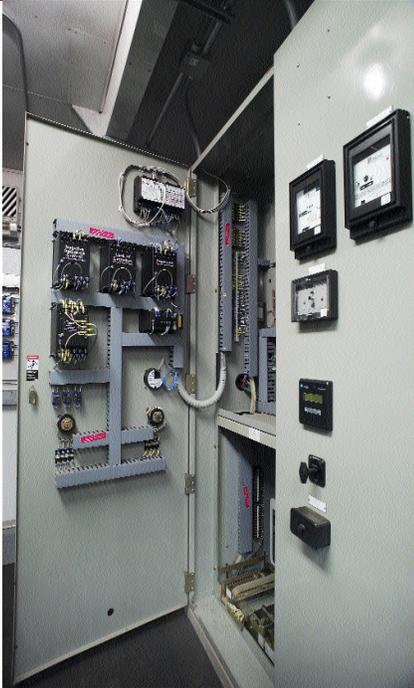
**Power meters from Rockwell Automation are installed on each of the facilities eight-diesel generators.**
