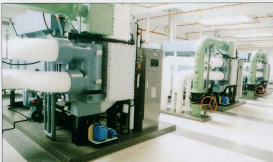
*Rockwell Automation integrated control system monitors and manages three McQuay gas absorption chillers used to cool buildings, and especially the data center, at Toyota's U.S. Headquarters.*
