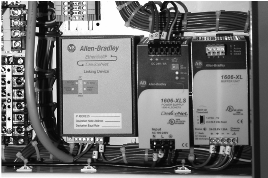
Figure 6.1 – LV Panel of Incomer with DeviceNet Power Supply
