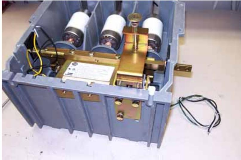
Figure 5 – Contactor (Front/bottom View)
