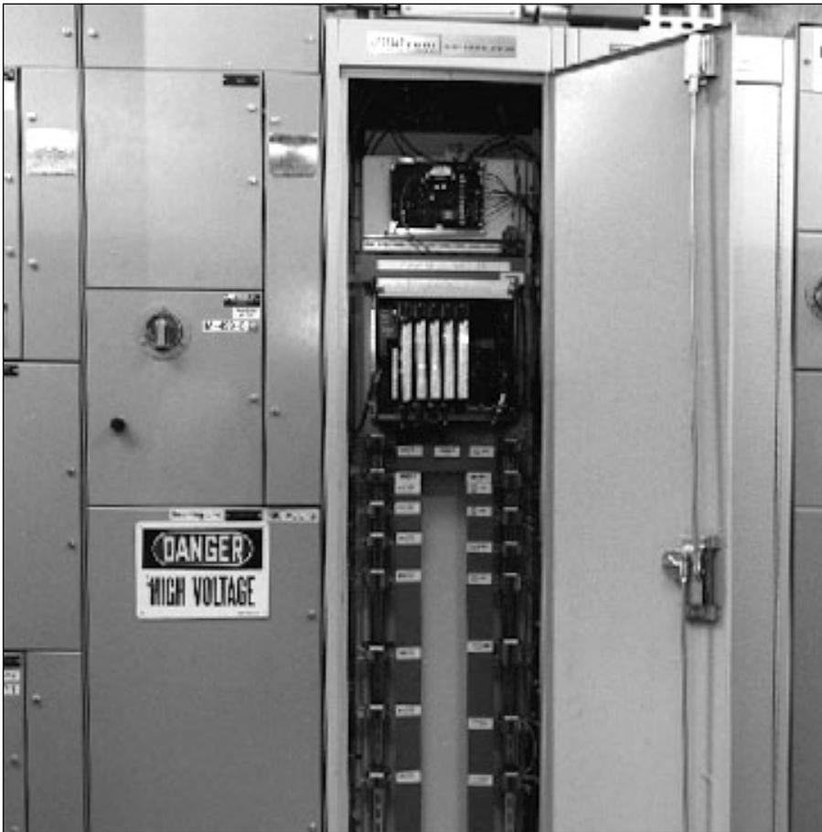
The need to resume operations quickly at Charlevoix meant that 1771 Remote I/O was installed in existing cabinetry, and connected to existing field wiring.
