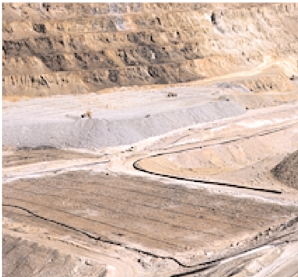
Two SLC controllers are used to monitor and control the pump that delivers the PLS from each heap pad to the SX processing area.
