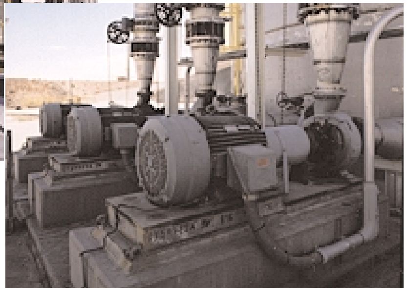
The process flow through solvent extraction trains (above) as well as bearing temperature on Reliance DutyMaster motors (right) are monitored with RSView software using data received via the ControlNet network.
