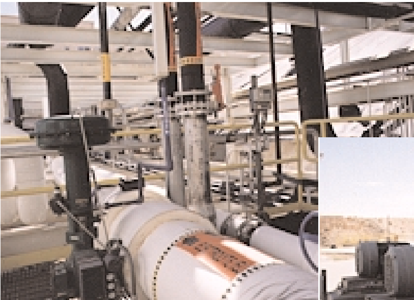
The process flow through solvent extraction trains (above) as well as bearing temperature on Reliance DutyMaster motors (right) are monitored with RSView software using data received via the ControlNet network.
