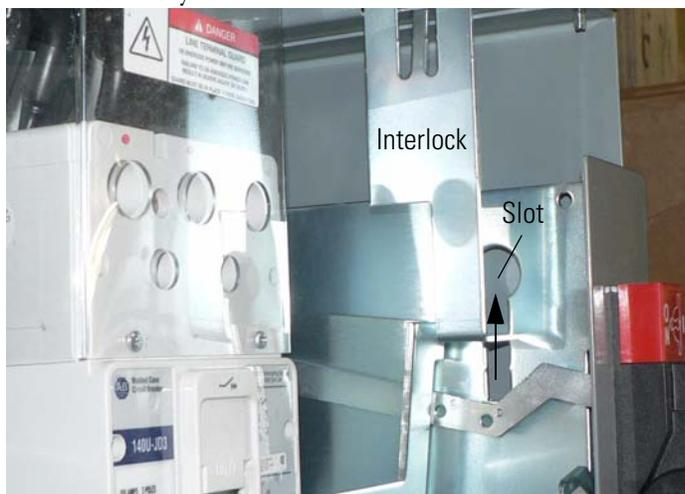
6. Tilt the bottom of the interlock towards the center of the unit.
