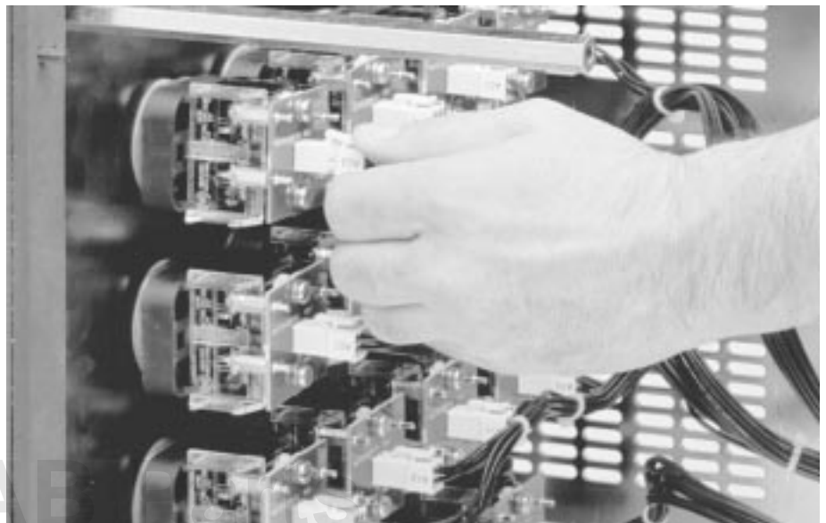
Figure G.1 Replacing 800T/H Push Buttons
